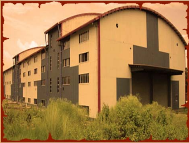
The newly built "Central Workshop"
